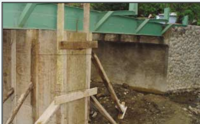
Construction of a bridge connecting Los Arroyos to the Community Complex
